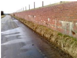
Figure 2 – Evidence of Seepage through Embankment Retaining Wall.
