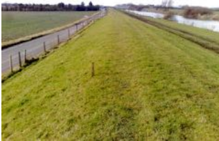
Figure 1 – Flood Defence Embankment on the River
