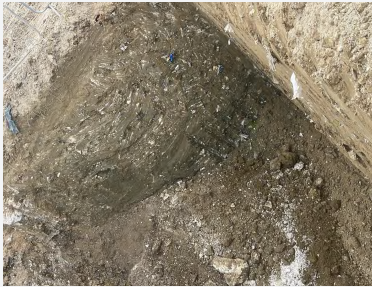
Soil mixed cell edge
