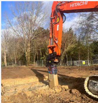
Soil Mixing in progress
